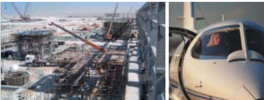
The Oryx gas-to-liquids plant under construction at Ras Laffan in Qatar.
