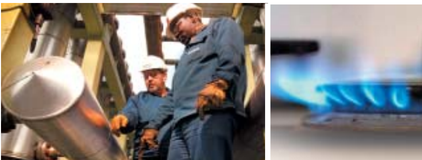
Two autothermal reformers for reforming natural gas were commissioned in 2004.
