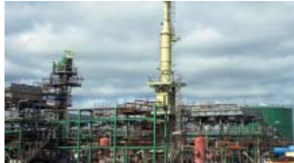
The central processing facility, under construction in Mozambique, was completed in 2004.
