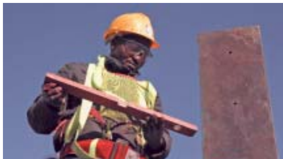
Work in progress for Project Turbo at Secunda in South Africa.
