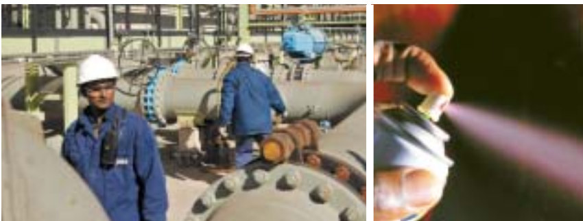
Site work progressing for the now completed acrylates complex.
